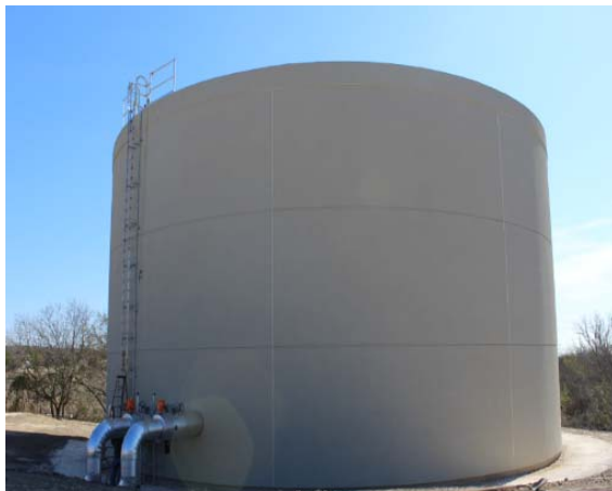
Alamo Community College – Northeast Lake View College (NLC) Thermal Energy Storage Tank. Similar TES Energy Assessment/design/installation mgmt. & Cx at NVC and PAC campuses (Demand response and load shift strategy). Planning, Design, Commissioning & const. Mgmt. by TEESI
