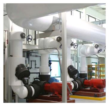
Under Phase 2- Additional cooling towers and a chiller were added to provide plant redundancy.
