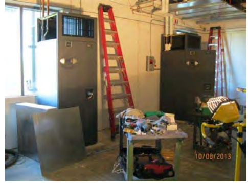
CRAH unit installation progressing in the data area.
