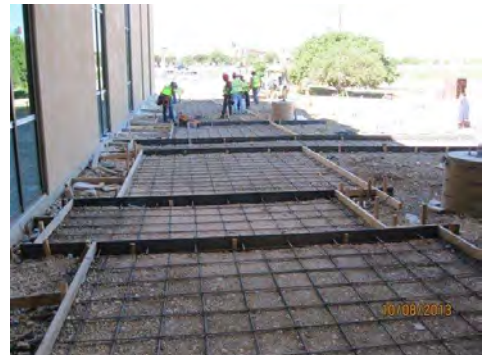
Flatwork progressing at the main lobby entry.
