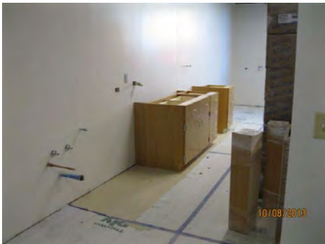
Casework progressing in the lab area.
