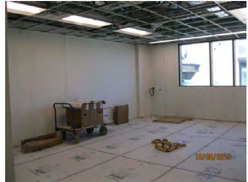
Interior finishes progressing in the BSL3 area.
