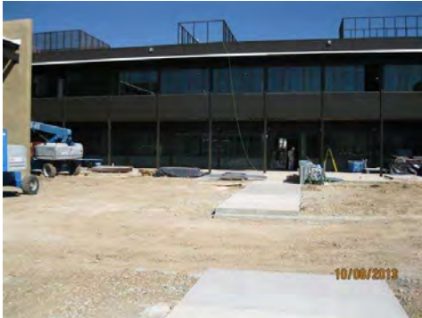
Work in the courtyard area progressing.
