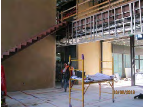
Work progressing in the main lobby.
