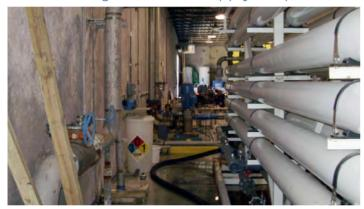
eHT provided planning, piloting, procurement, design and construction services for expansion of the existing surface water treatment plant (WTP), including addition of a second RO system consisting of two trains with a total capacity of 600 gpm. The RO system permeate was blended with the pretreated effluent from the Intermediate Pump Station. Treated water from the RO membrane unit was combined with pretreated effluent, disinfected, stored, and pumped to the existing distribution system.
