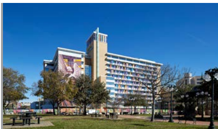
CHRISTUS Health System, Children's Hospital; $110,807,128; 400,000 SF; San Antonio, TX
