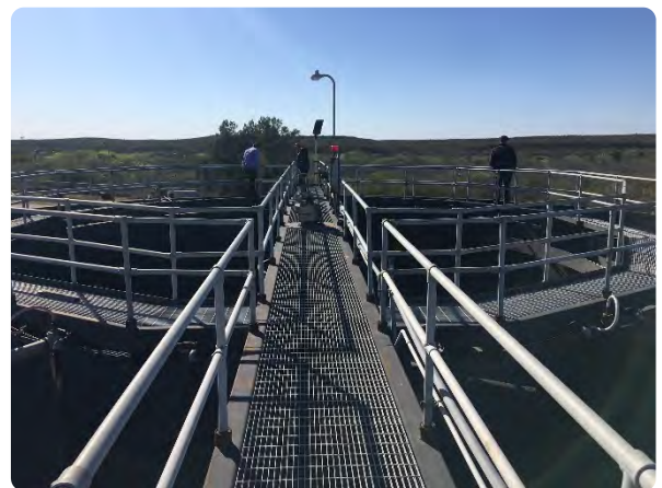
The ESG Team on-site at Rio Bravo WWTP
