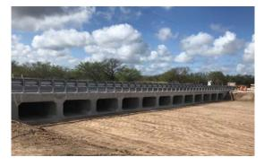
Las Lomas Culvert & Roadway Improvements – Surveys, Plans, Specifications and Construction Oversight were prepared for Webb County to construct two (2) bridge class culverts and 2,600 feet of new roadway in the Las Lomas Colonia in Eastern Webb County. The project was constructed by Webb County Road and Bridge force and US Army crews. This project is nearly complete.
