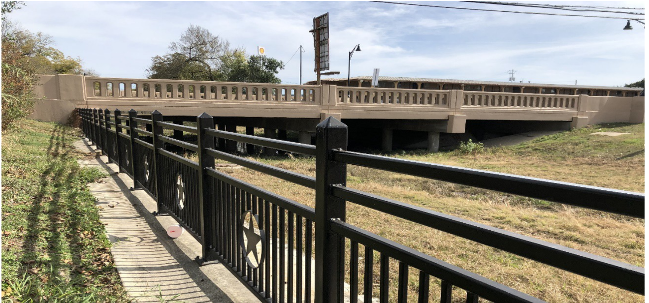
Guadalupe Street Bridge, San Marcos
