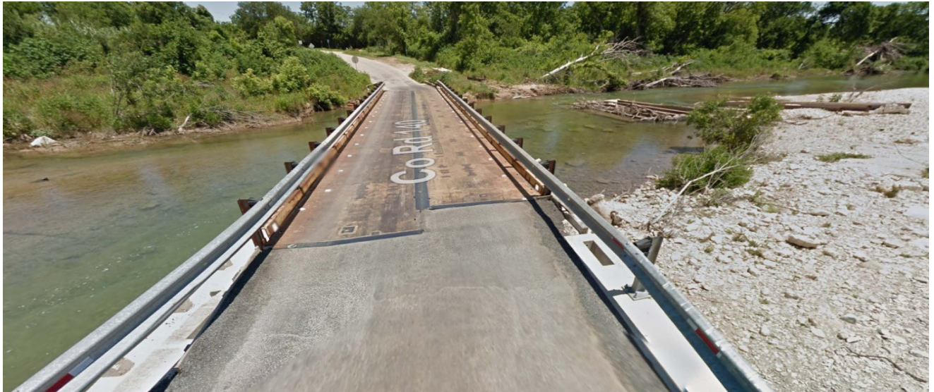
Temporary Rail Car Bridge at Post Road
