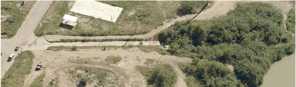
Figure 3—Centeno Lane outfall into the Rio Grande showing the outfall chute has been undermined. Roughly 400 cfs pass through the Centeno Lane outfall at the red line shown in 3.
