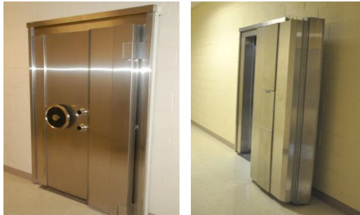
The Level 5 door of the Long-Term Storage Vault (same model used for each vault).
