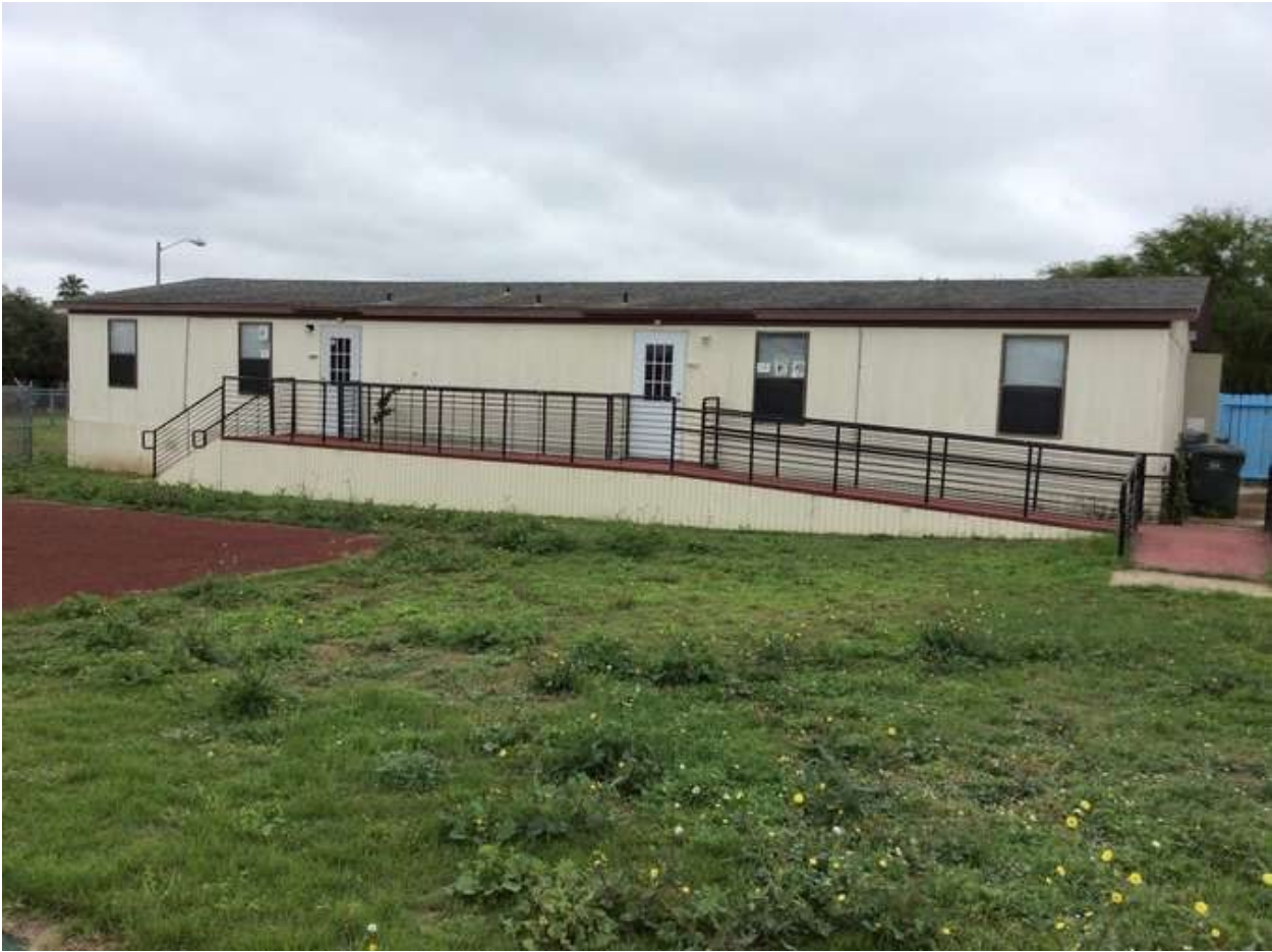
BUILDING TWO – FRONT VIEW
