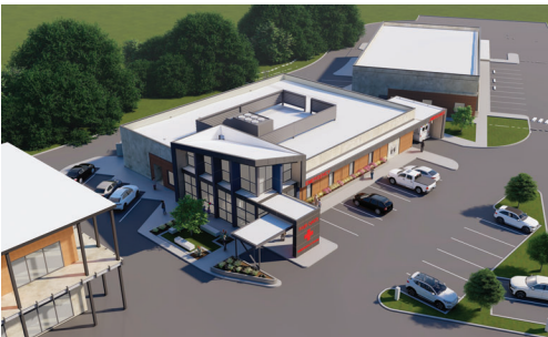
Fair Oaks ER-Under Construction
