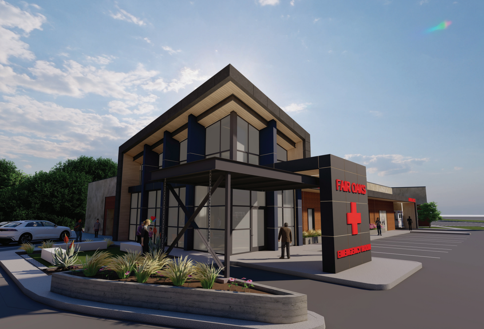
FAIR OAKS ER-UNDER CONSTRUCTION
