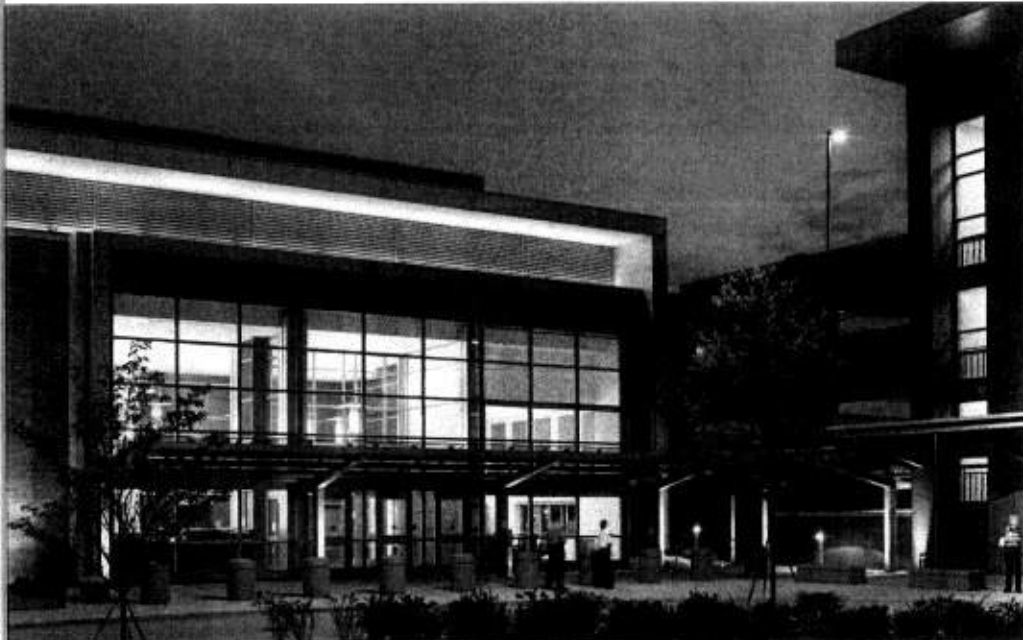
Cover: U.S. Federal Courthouse, Laredo, Texas; Denton County Law Enforcement Master Plan, Denton, Texas Above: Wake County Jail Phase 2, Raleigh, North Carolina
