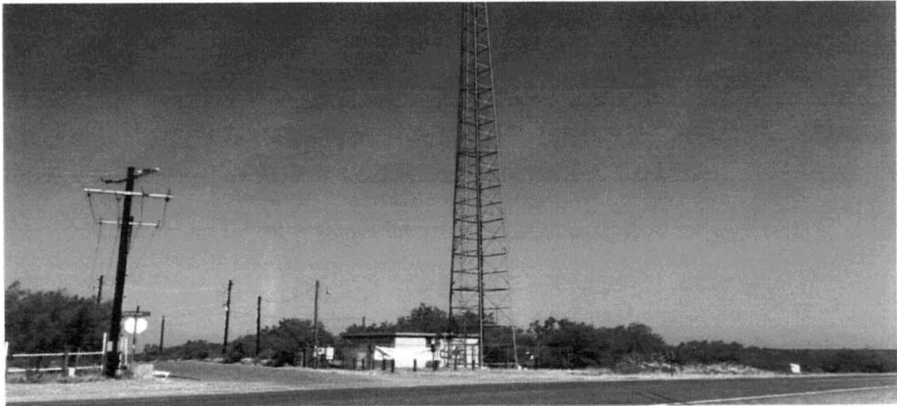
Future Site of Los Botines Fire Station – at the intersection of HWY 83 N. & San Juan Rd.
