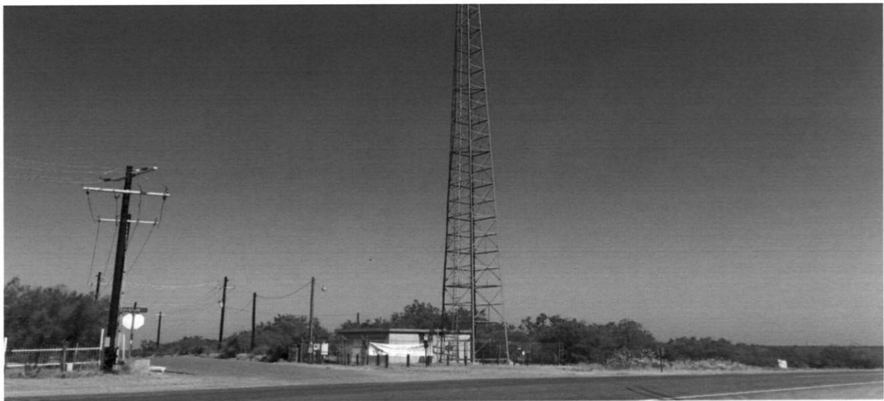
Future Site of Los Botines Fire Station– at the intersection of HWY 83 N. & San Juan Rd.
