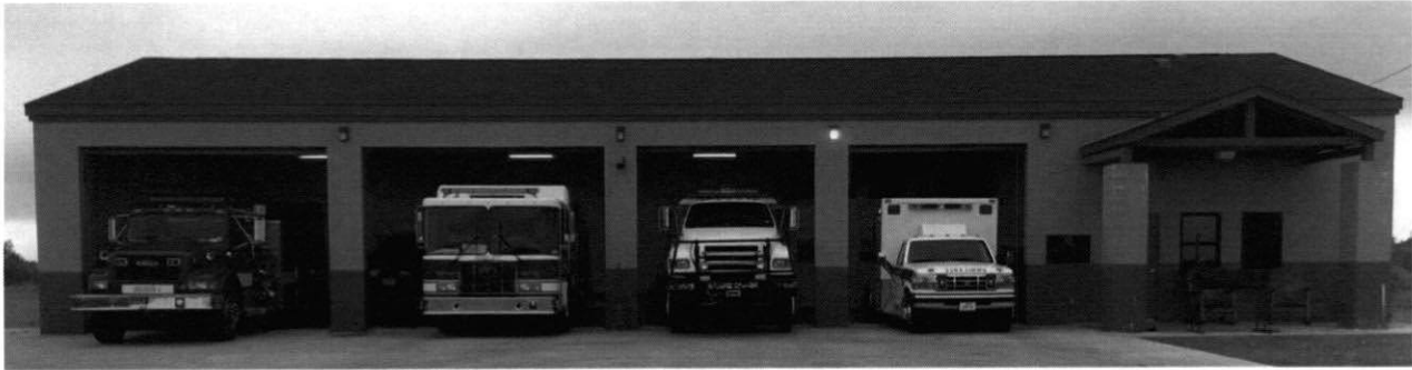
Webb County- Quad City Fire Station - Bruni, TX
