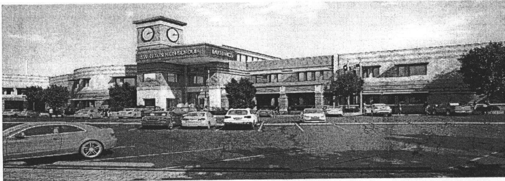
Laredo ISD - Nixon High School, 200,000 SF replacement campus (MEP by TEESI)
