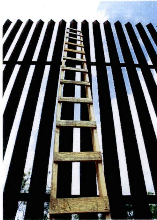
Ladder on South Texas border wall
